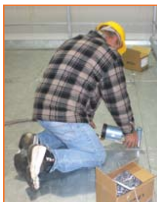
Steel floor fastening
