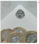
Placing fasteners in tight corners makes access for impulse tampering more difficult.
