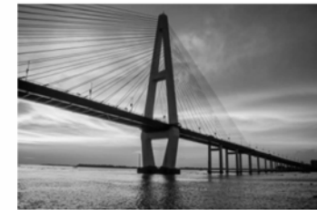
Steel bridge construction
